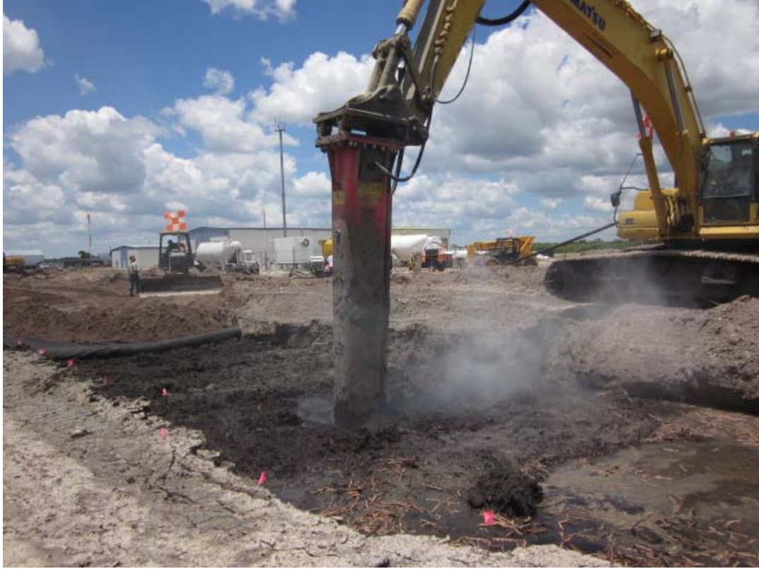
Figure 1.2 Dry soil mixing showing clouds of powdered cement injected below ground.
