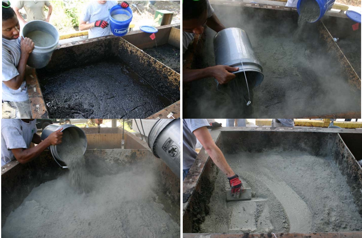
Figure 4.29 Introducing dry cement to soil.
