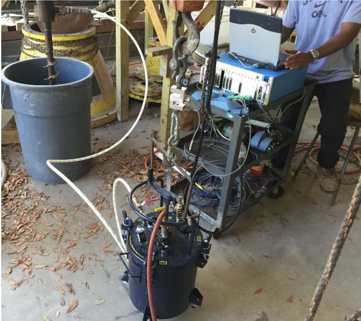
Figure 4.10 Grout calibration setup.
