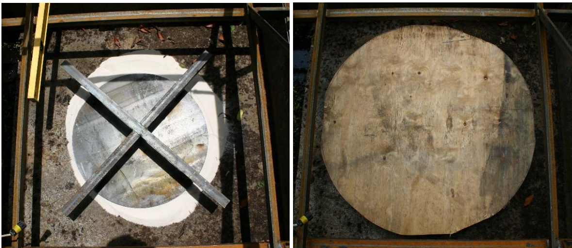
Figure 4.34 Bearing plate assembly with plywood.
